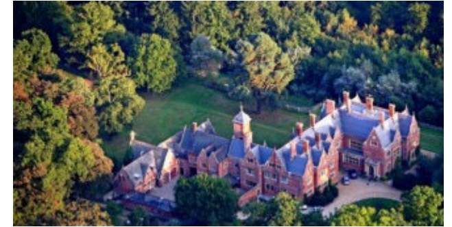
MANOR HOUSE, DAUNTSEY'S SCHOOL, WEST LAVINGTON, Nr DEVIZES
